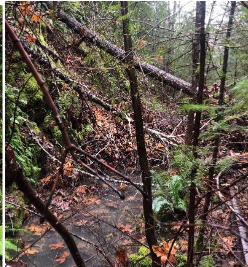
Photo 4 MP 151.6 poor drainage
