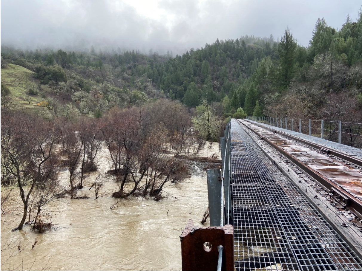
Photo 16 Bridge 151.99 Outlet Creek overflowing banks
