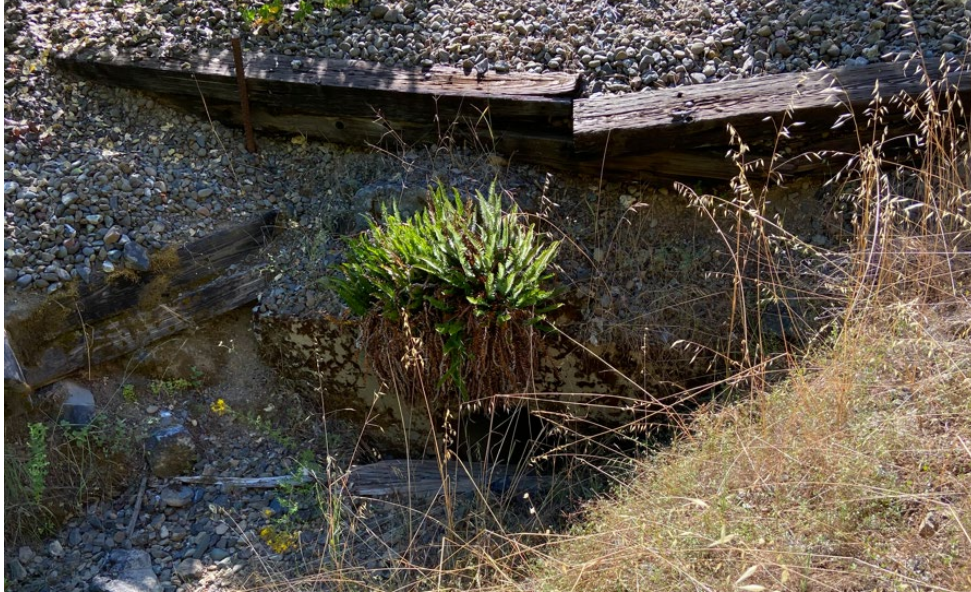
Photo 9 Example of ineffective headwall
