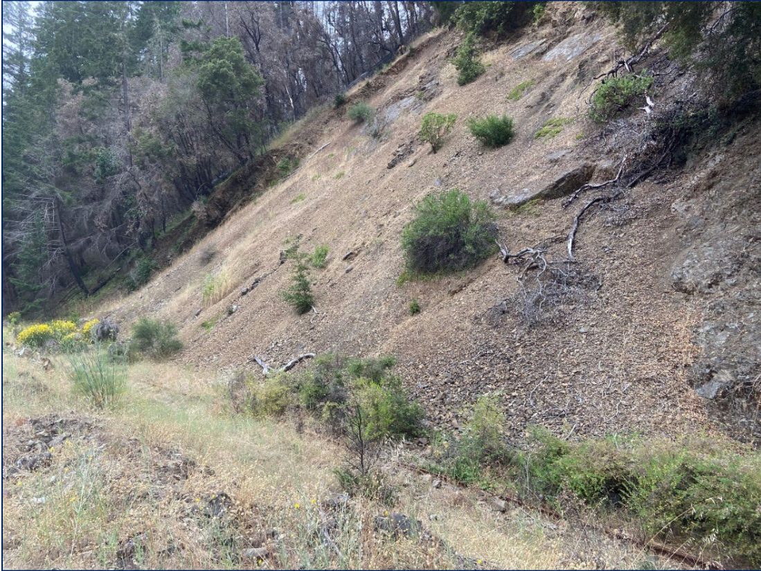
Exhibit 4-4 - Photo 95 – Highly fractured siltstone and mudstone interbedded with blocky sandstone exposed on slope at approx. MP 146
