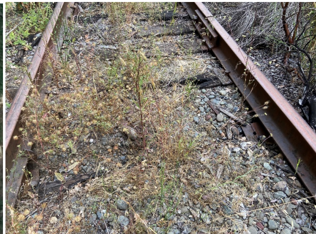
Photo 14 Fire damaged track and substandard ballast.
