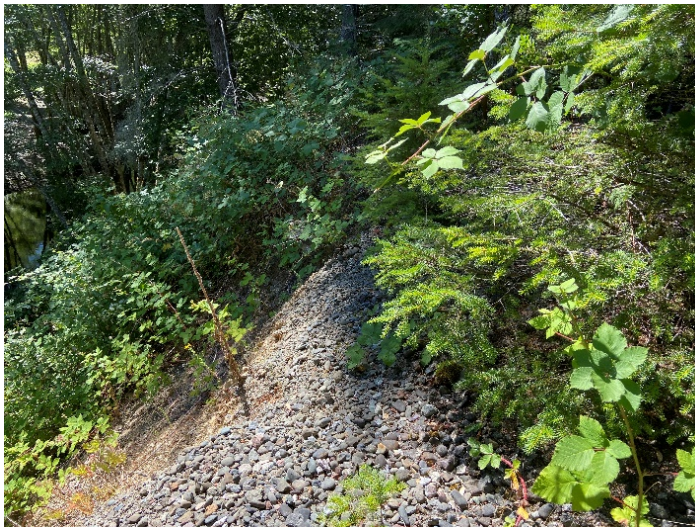
Photo 3 MP 151.6 steep slope at Outlet Creek.
