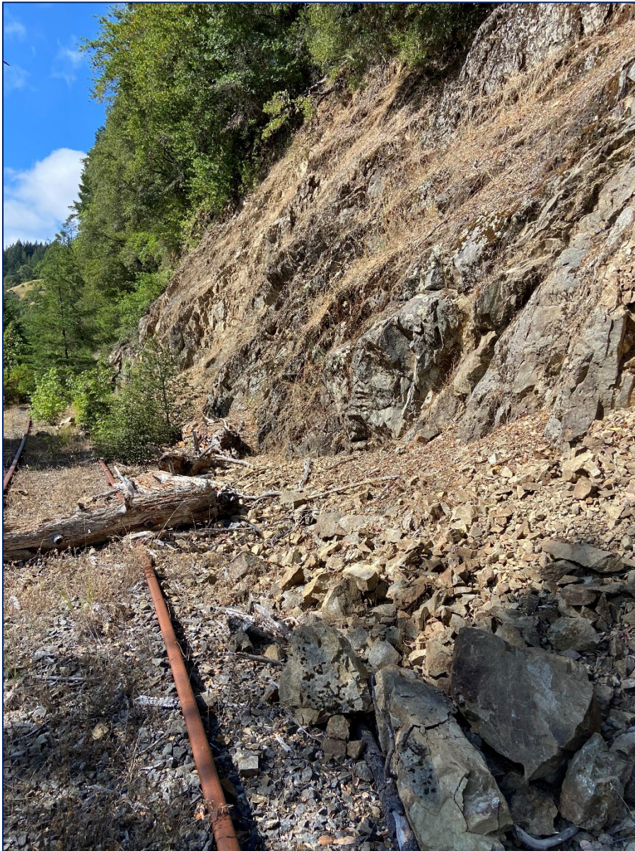
Exhibit 4-5 - Photo 15 – Folded and fractured sandstone and siltstone rock slope at approx. MP 151.87
