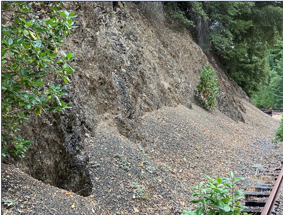
Exhibit 4-3 – Photo 65 – Fragments of highly fractured siltstone and mudstone raveling from rock slope at approx. MP 147.3
